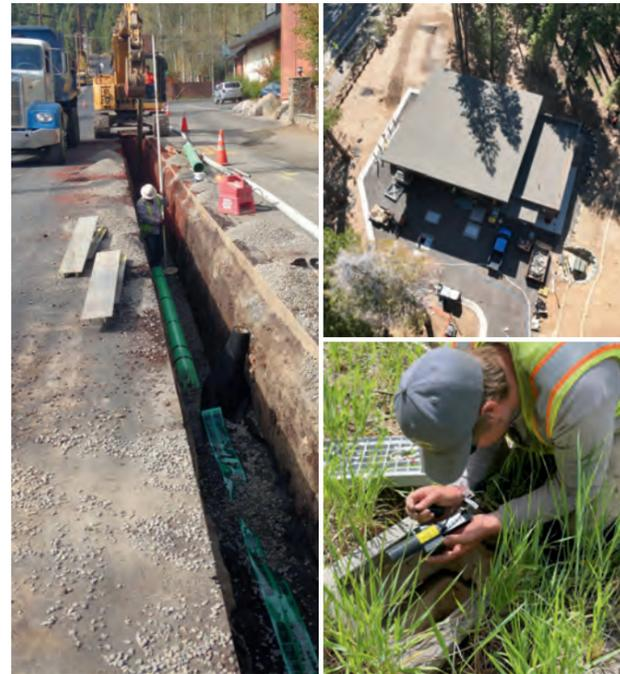
Left: Crews install new sewer main. Top right: An aerial view of the new West Lake Tahoe Water Treatment Plant. Bottom Right: TCPUD staff install a new SMART water meter.
